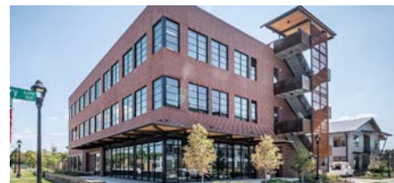
101 Nursery Lane - The second phase of the Nursery Lane Office Park, developed by Fort Capital. This 19,902 SF office and retail building was named the first-ever "Dream Office" by FW Inc. magazine and features the latest design trends and amenities.
